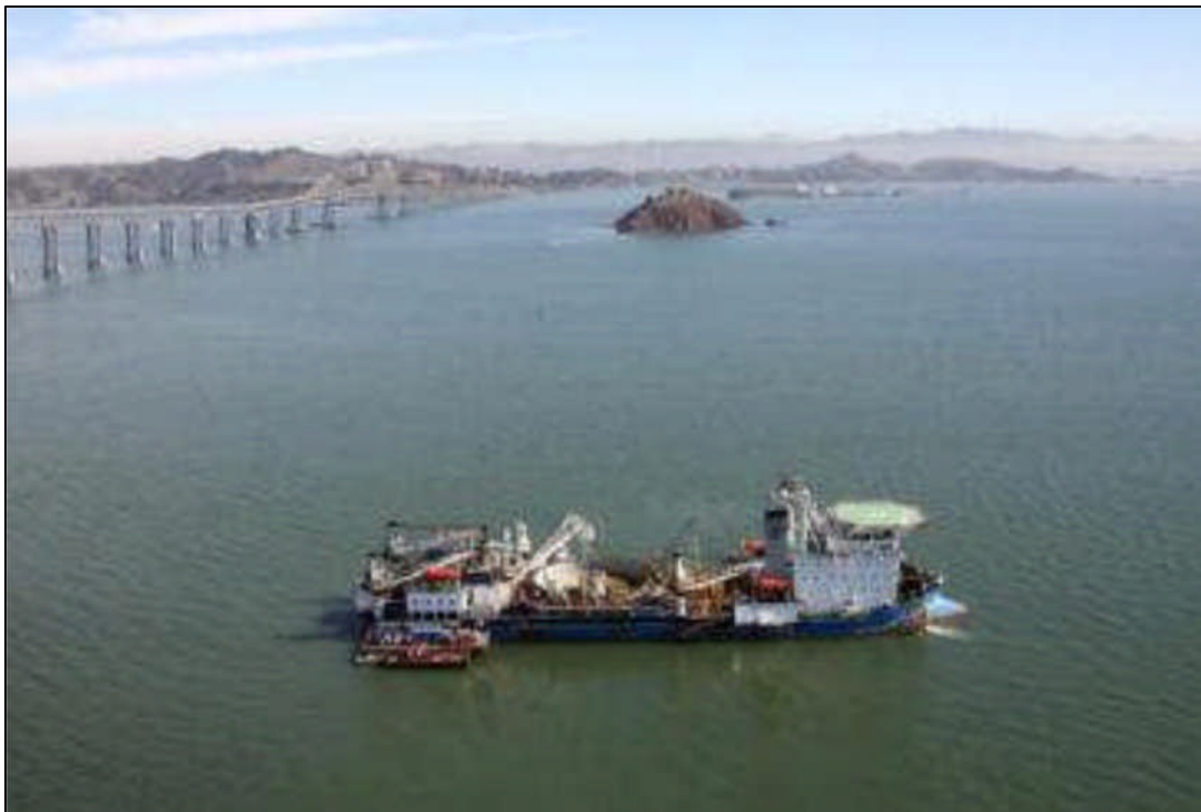
Cable Laying vessel - Giulio Verne
